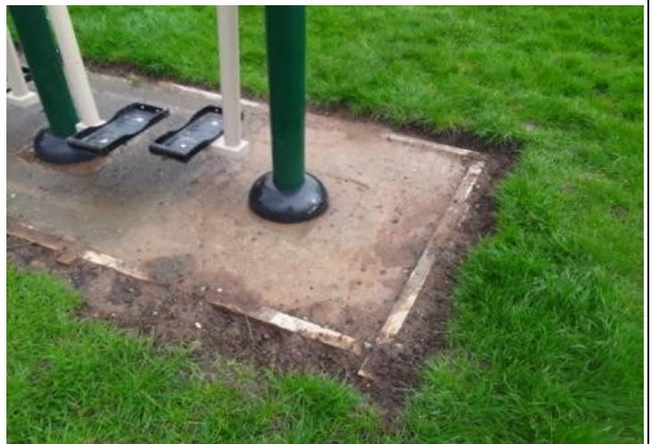
**Finding:** There are trip hazards at the edges of the surface **Action:** Reinststate surrounding surface levels to remove the trip points
