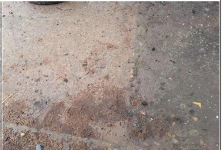
**Finding:** Whilst not a safety concern, the client has pointed out that there are some inconsistencies within the finished concrete (Some of the surface is pre-existing)
