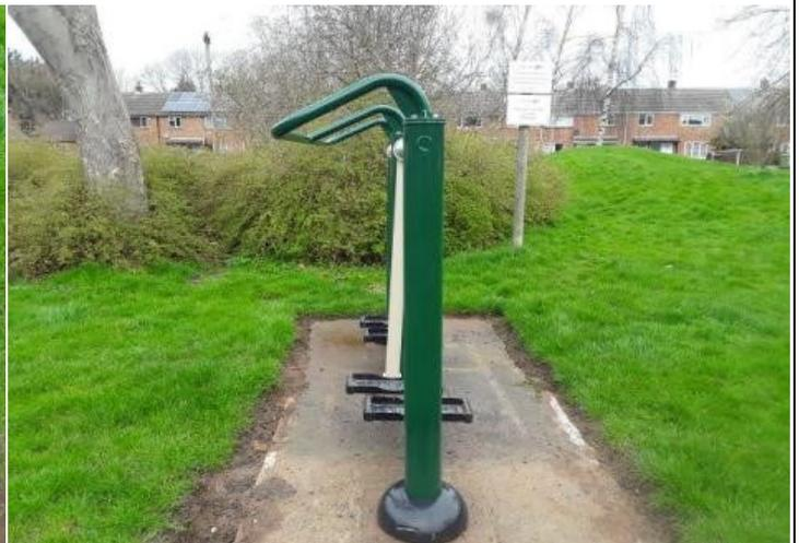
**Finding:** The posts are misaligned and the footplates are with each other at rest
