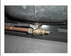
**Viessmann 6182 Vitovalor PT2** in the boiler room, drain valve at the base of the Calorifier
