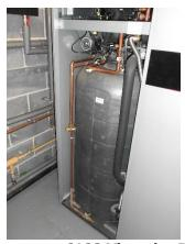
Viessmann 6182 Vitovalor PT2 in the boiler room, 220L hot water tank
