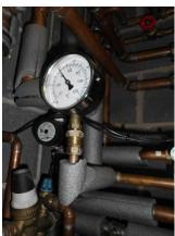
**Viessmann 6182 Vitovalor PT2** in the boiler room, temperature gauge on the flow
