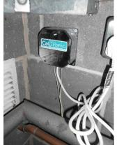
Caltronic electronic scale inhibitor on the mains in boiler room
